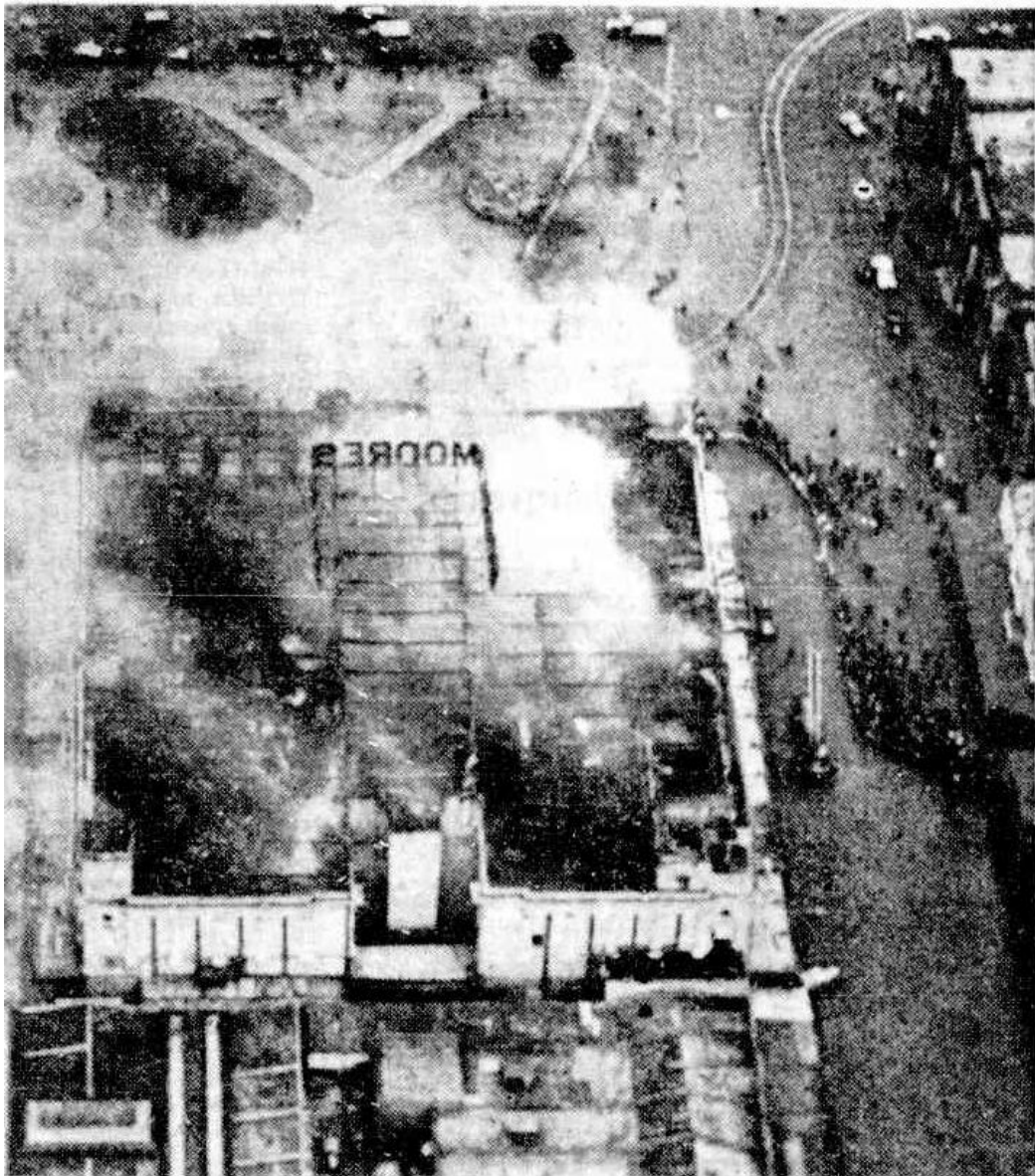
TODAY'S AIR PICTURE of last night's big fire scene shows smoke still pouring from the building.
